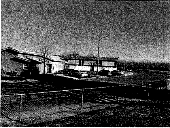
Future access on McKeehan Drive facing south
