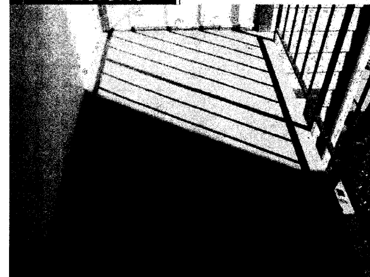
Stair landing surface at Unit A1
