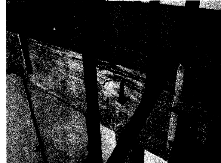
Wood decay at beam above support post at Unit B11. Note weathering and warping of landing sheathing.
