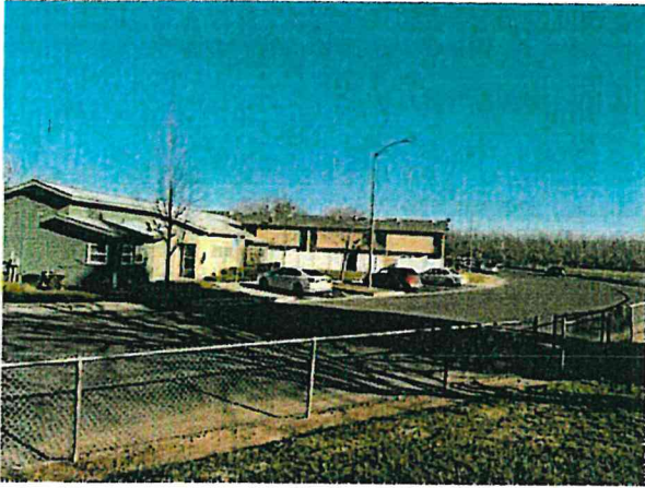
Future access on McKeehan Drive facing south
